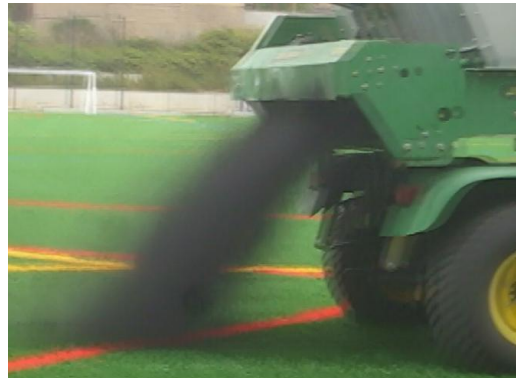
spreading tire crumb on top of plastic turf
